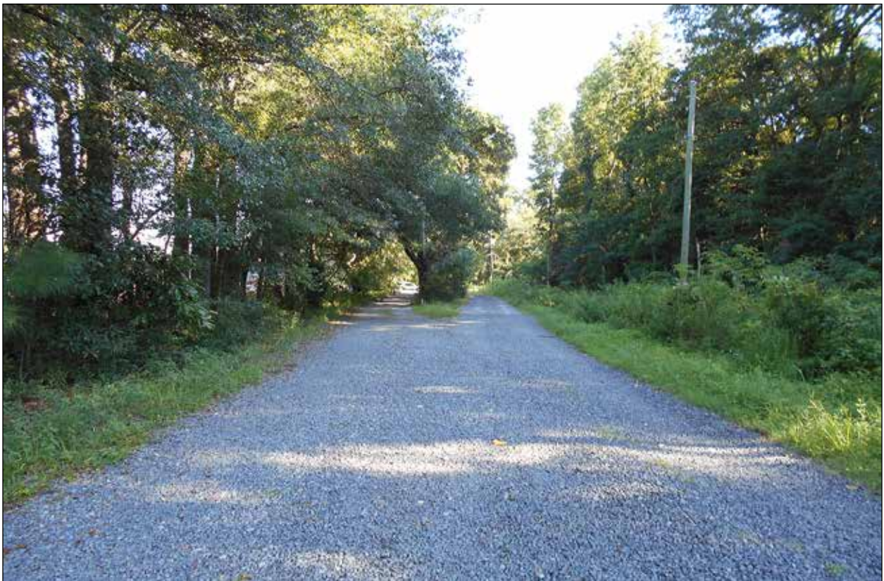
Figure 1.3 Typical views of the Clements Ferry Road Widening Project: Fogarty Lane, facing north (top); Oakview Lane, facing north (bottom).
